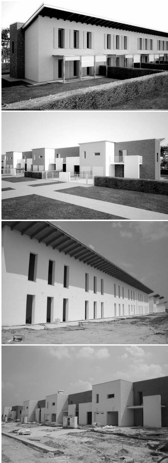
Figure 2: Two renderings (above) compared with photos of the last building during construction (below).
